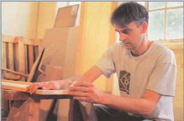
Above Hand-sanding an edge - there are times when machine sanding isn't possible Right A random orbital sander will give very good results
