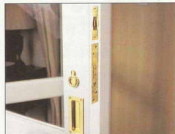
The neatly installed brass fittings
